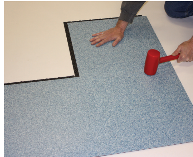
LOCK SEAM using a simple mallet
