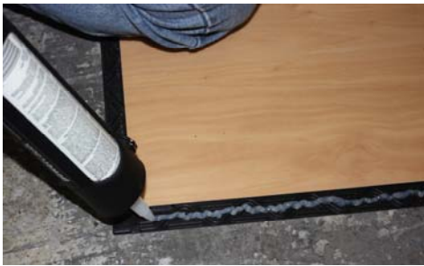
Apply 1/8" Bead of Sealer Along Center of Exposed Tabs
