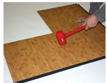
LOCK SEAM using a mallet
