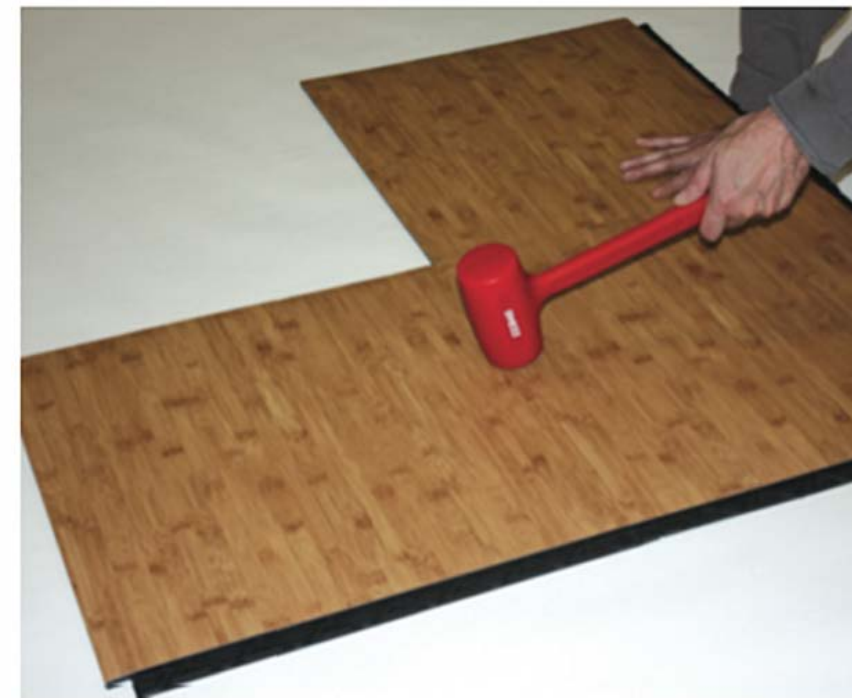
LOCK SEAM using a simple mallet
